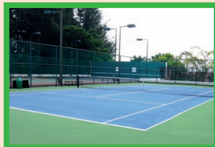
Courts 1 & 2 – After renovation
